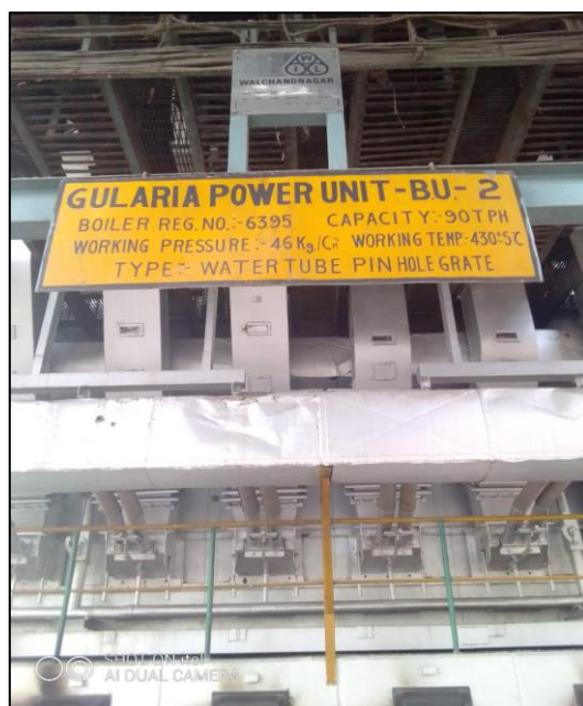
Figure 3: An image of boiler installed in the plant
